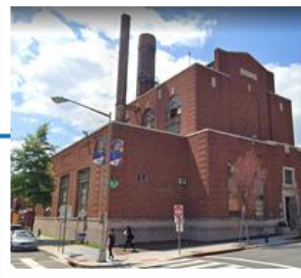
Steam Plant Modernization 2023
