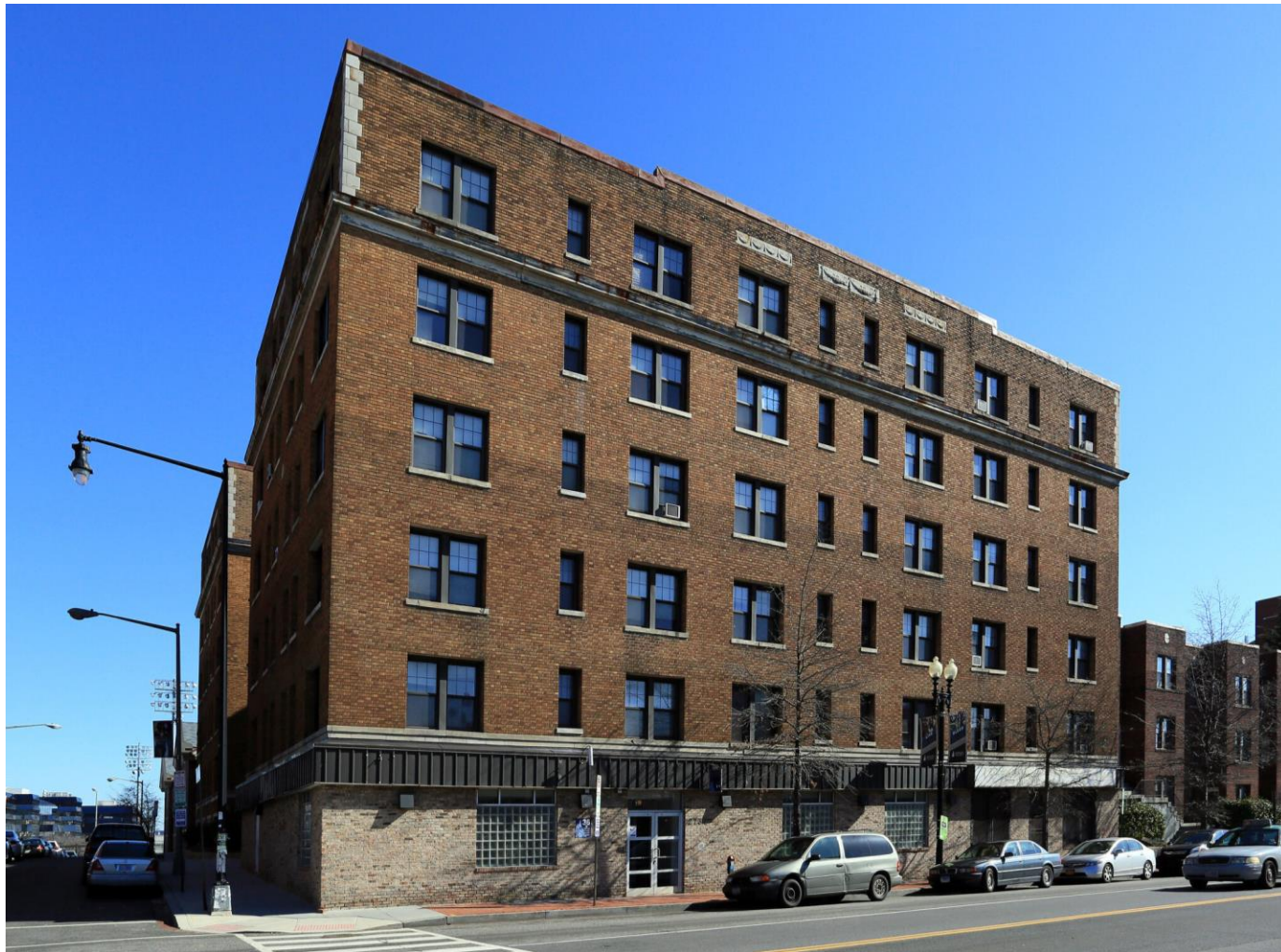
Existing conditions, prior to work commencement
