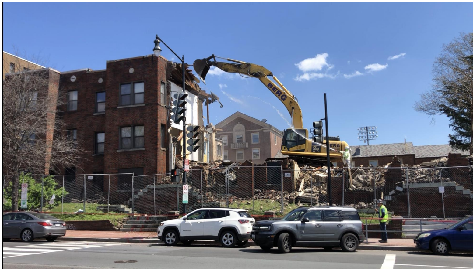
Demolition, currently under way at Effingham Apartments
